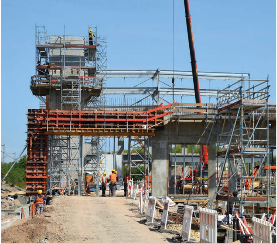
Mobility centre, D-Karlsruhe; Züblin, construction engineering Karlsruhe
