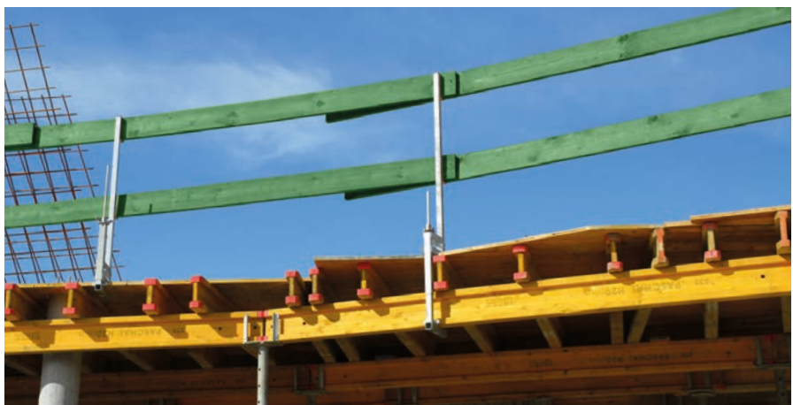
Use on slab formwork with clamping piece
