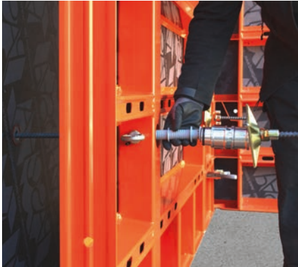
For single-sided anchoring, the tie rod together with the tube, the guide bushing and plate with ball-andsocket joint are turned into the clamping unit of the outer formwork.
