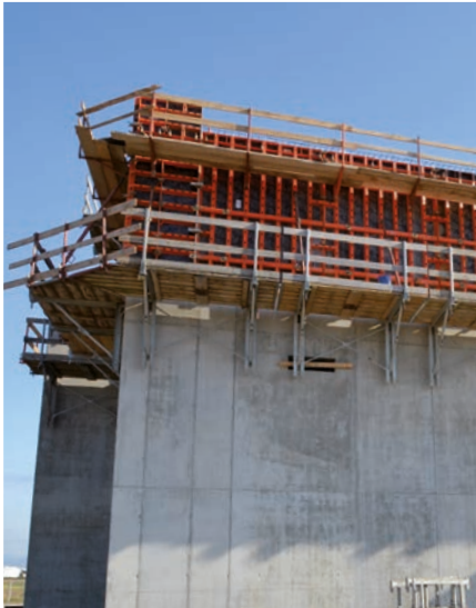
Climbing platform KBK 180 Work and jacking scaffold, which comes fully assembled and ready to use on-site.
