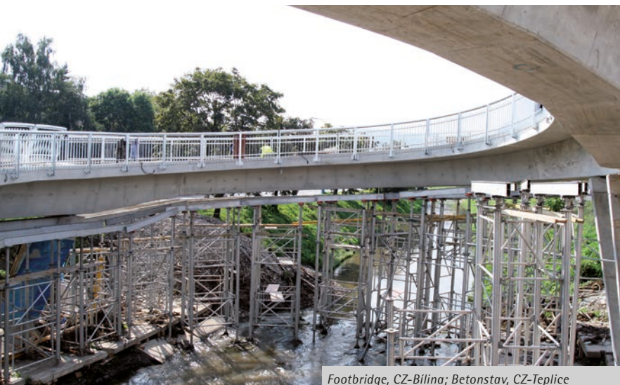
Footbridge, CZ-Bílina; Betonstav, CZ-Teplice
