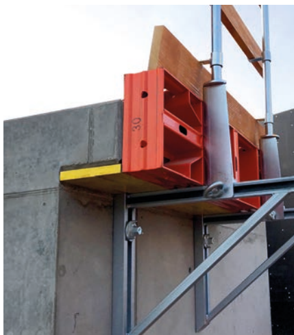
For concreting the brackets, the stop can be adjusted by up to 50 cm.
