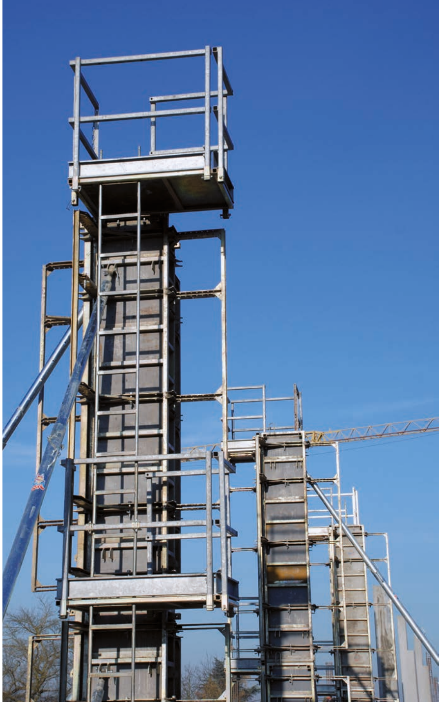
Supermarket, D-Kenzigen; Singler Bau, D-Hofstetten
