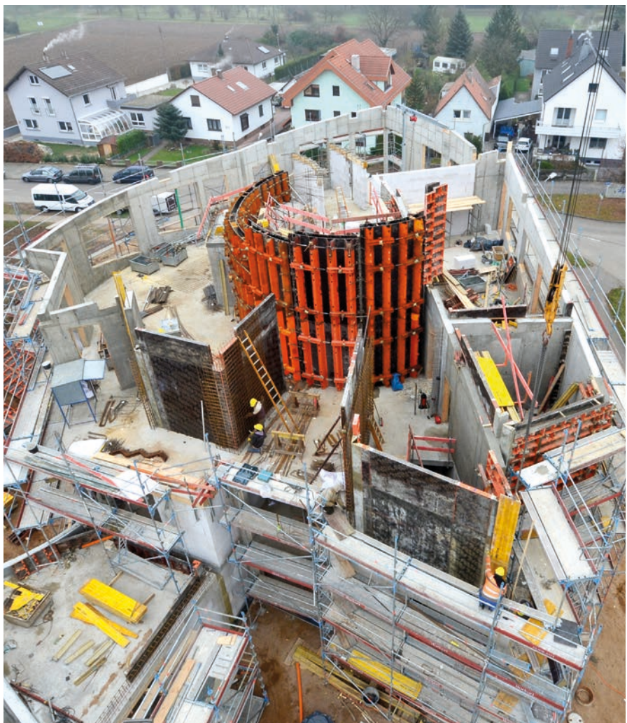
Parzival school, D- Karlsruhe; Weisenburger Bau GmbH
