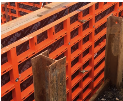
Clamping unit flush mounted in the panel frame
