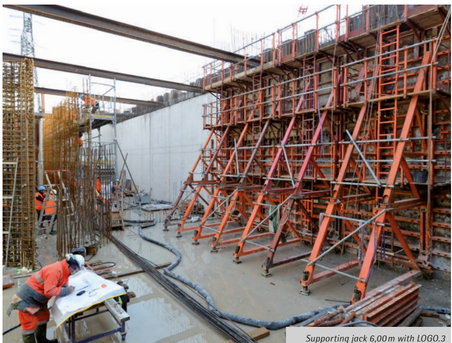
Fish ladder, F- Rohrschollen; GTM-HALLE, F-Schiltigheim
