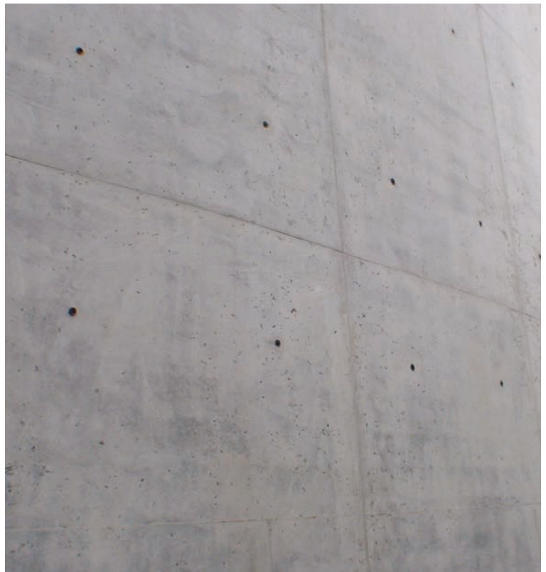
Top class concrete surface
