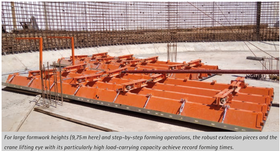
Crane lifting eye KBT
