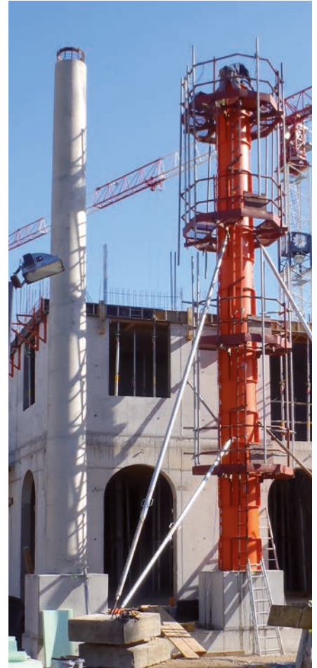
Circular columns with conical shape; mounted working platforms with ladders as access serve for security during forming, dismantling and pouring concrete. Hotel „Bell Rock“ Europa-Park Rust; Implenia Bau GmbH, D-Rümmingen
