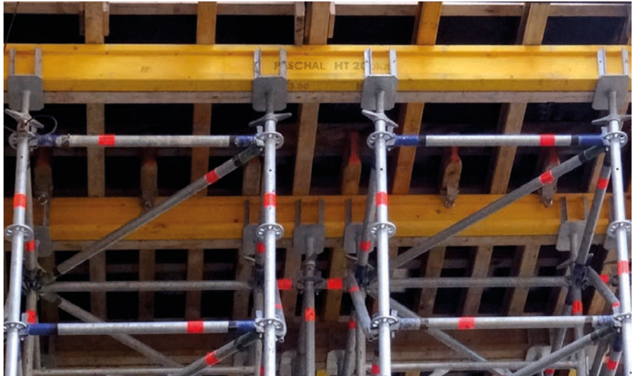
Superstructure with spindle, support beam and cross-beam
