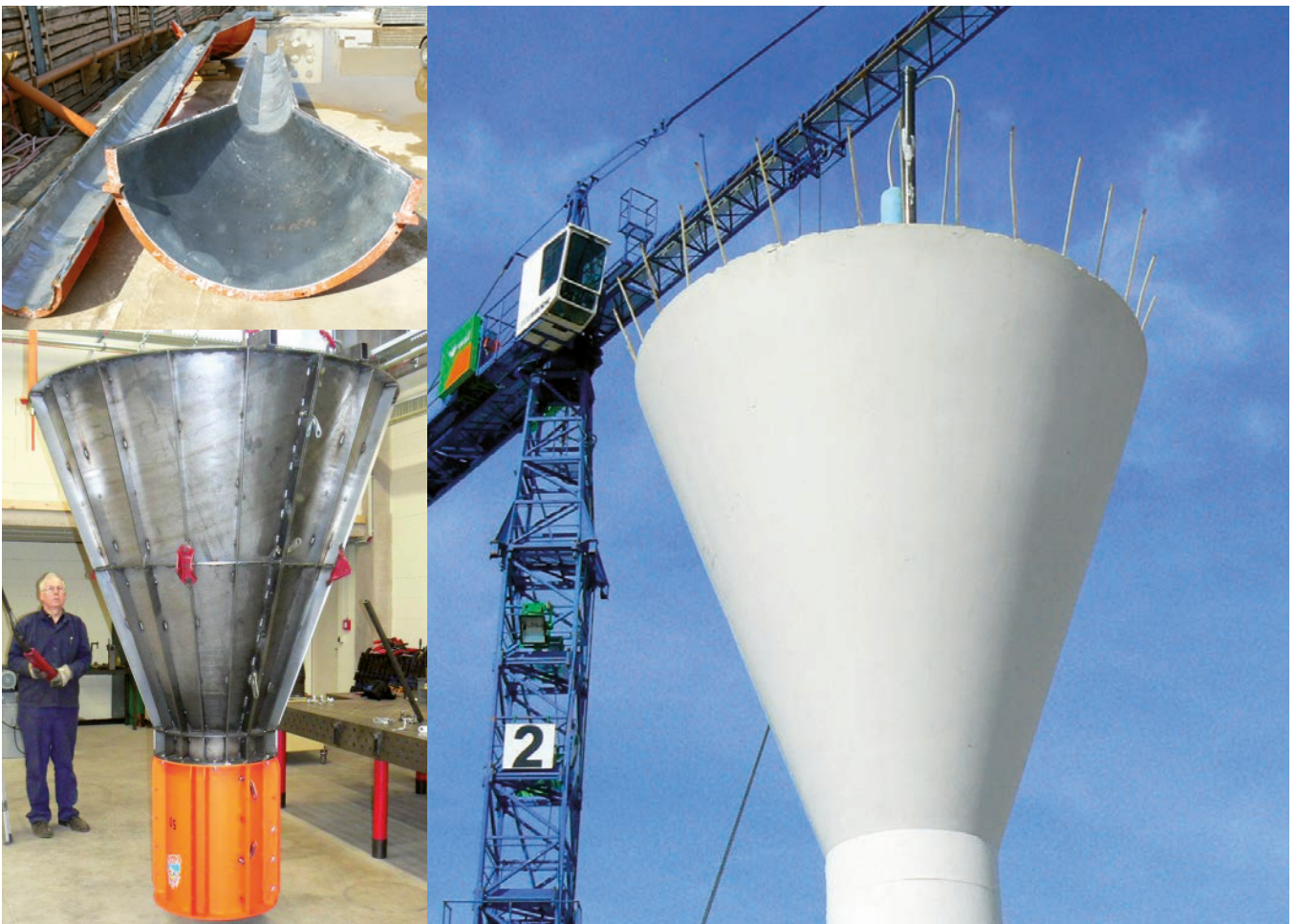
Mushroom head formwork – National theatre Darmstadt (white concrete)
