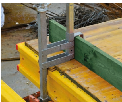
Lateral protection clamping piece and protection fence
