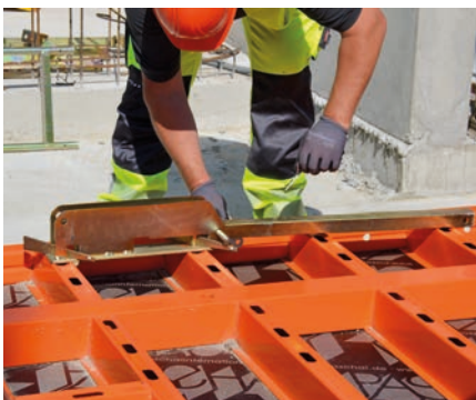
Ready-assembled units of formwork with working platforms are ready for transport.
