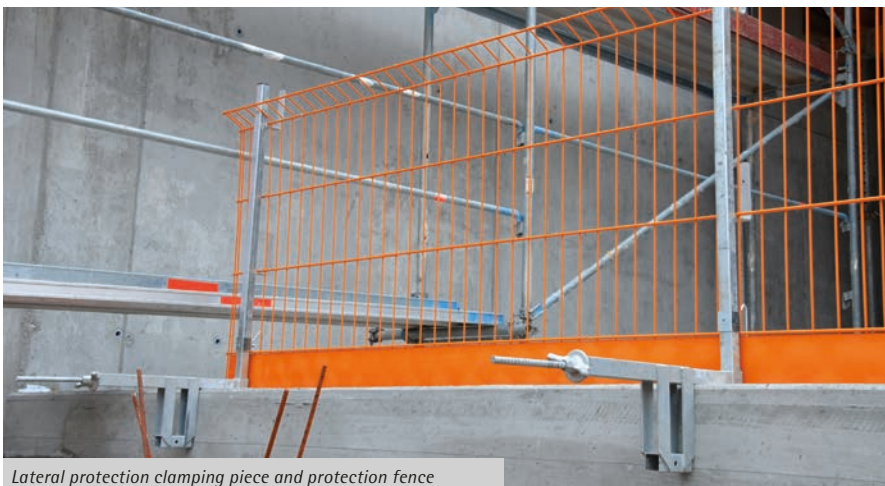
Lateral protection clamping piece and protection fence
