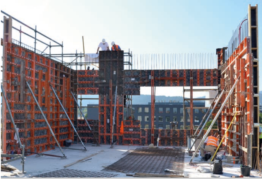
IMBIT research building, University Freiburg; Implenia AG
