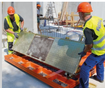
Ready-assembled units of formwork with working platforms are ready for transport.
