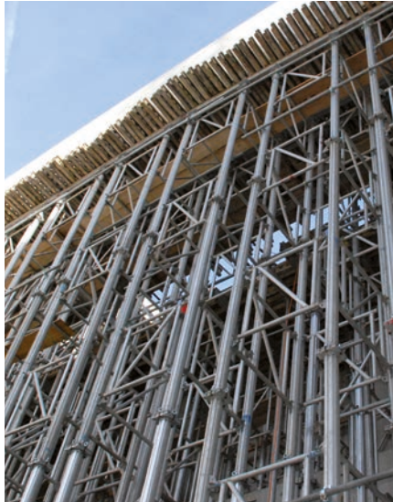
Aluminium shoring system GASS
