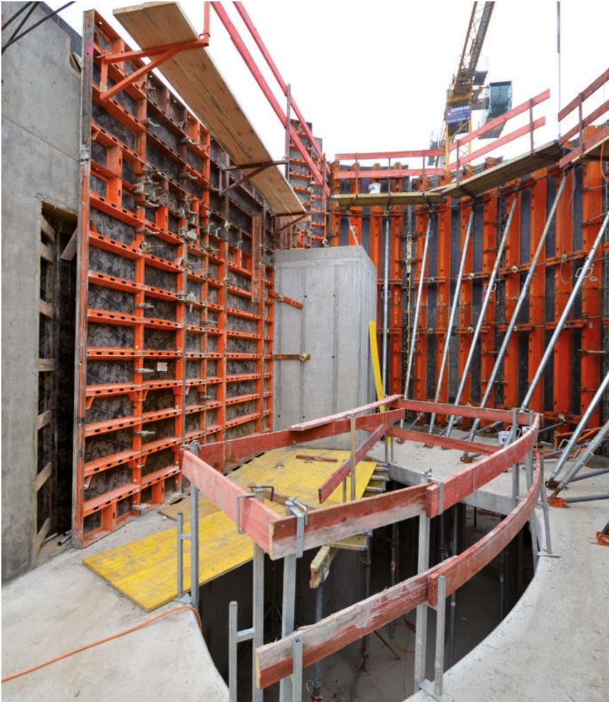
Parzival school, D- Karlsruhe; Weisenburger Bau GmbH
