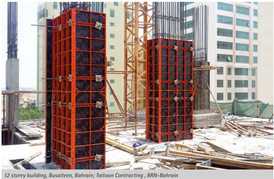
12 storey building, Busaiteen, Bahrain; Taitoon Contracting, BRN-Bahrain
