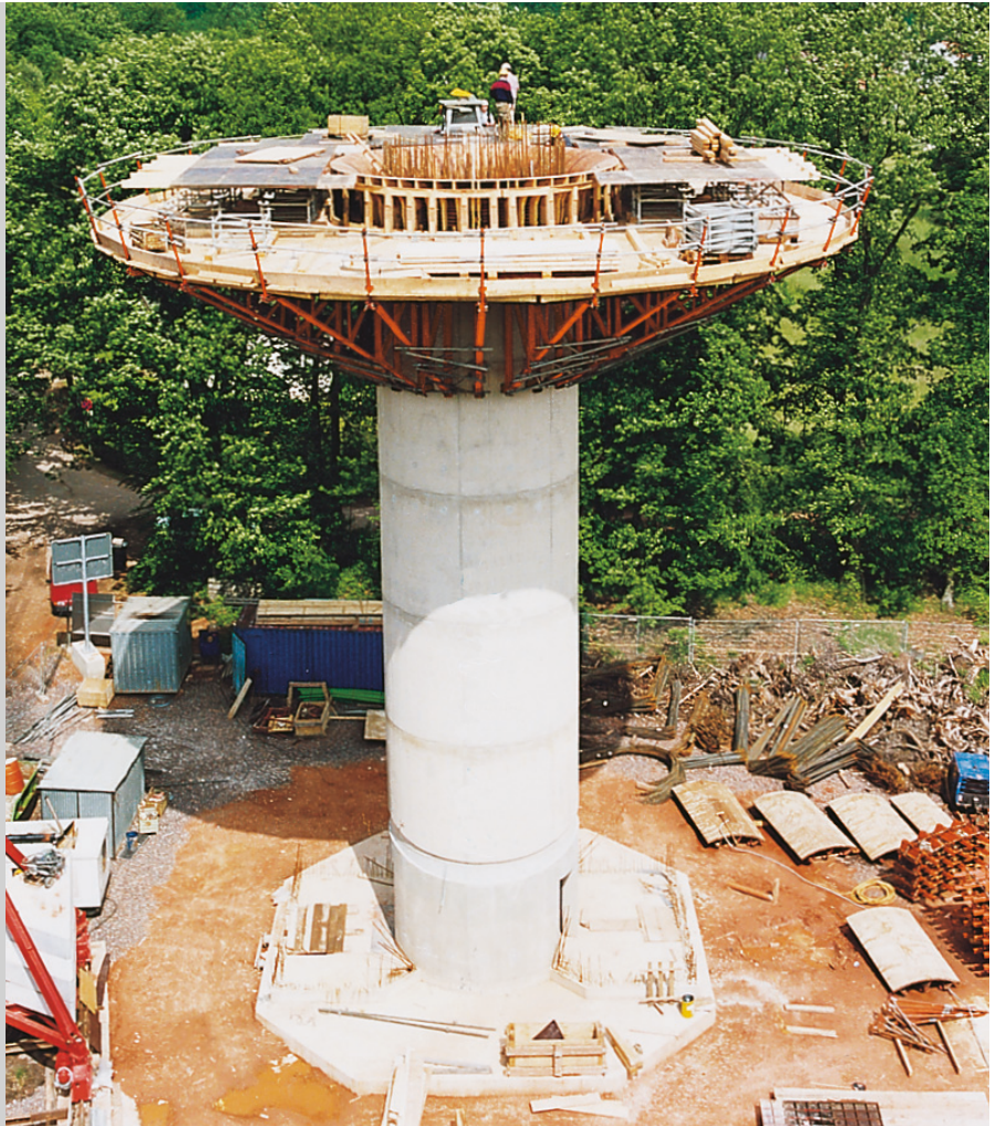
Water tower, Lauterbach; Walter Bau AG, Kirkel-Limbach
