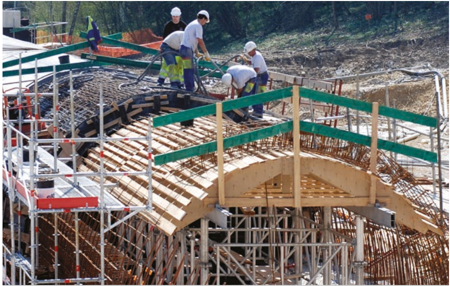
Vault formwork, F-Rougement; GTM, F-Les Magny
