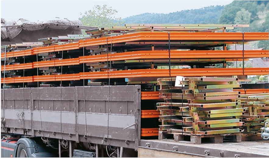
Ready-assembled units of formwork with working platforms are ready for transport.
