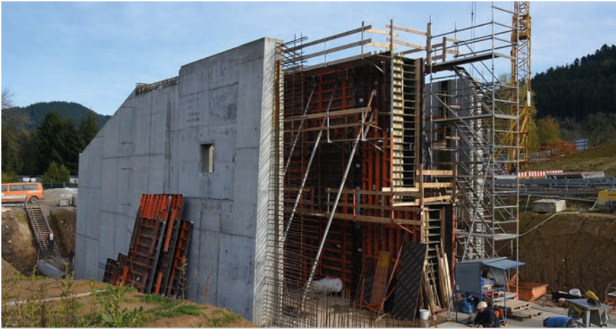
Cellar in residential building, D-Ergolding; Lachermeier GmbH, D-Ergolding
