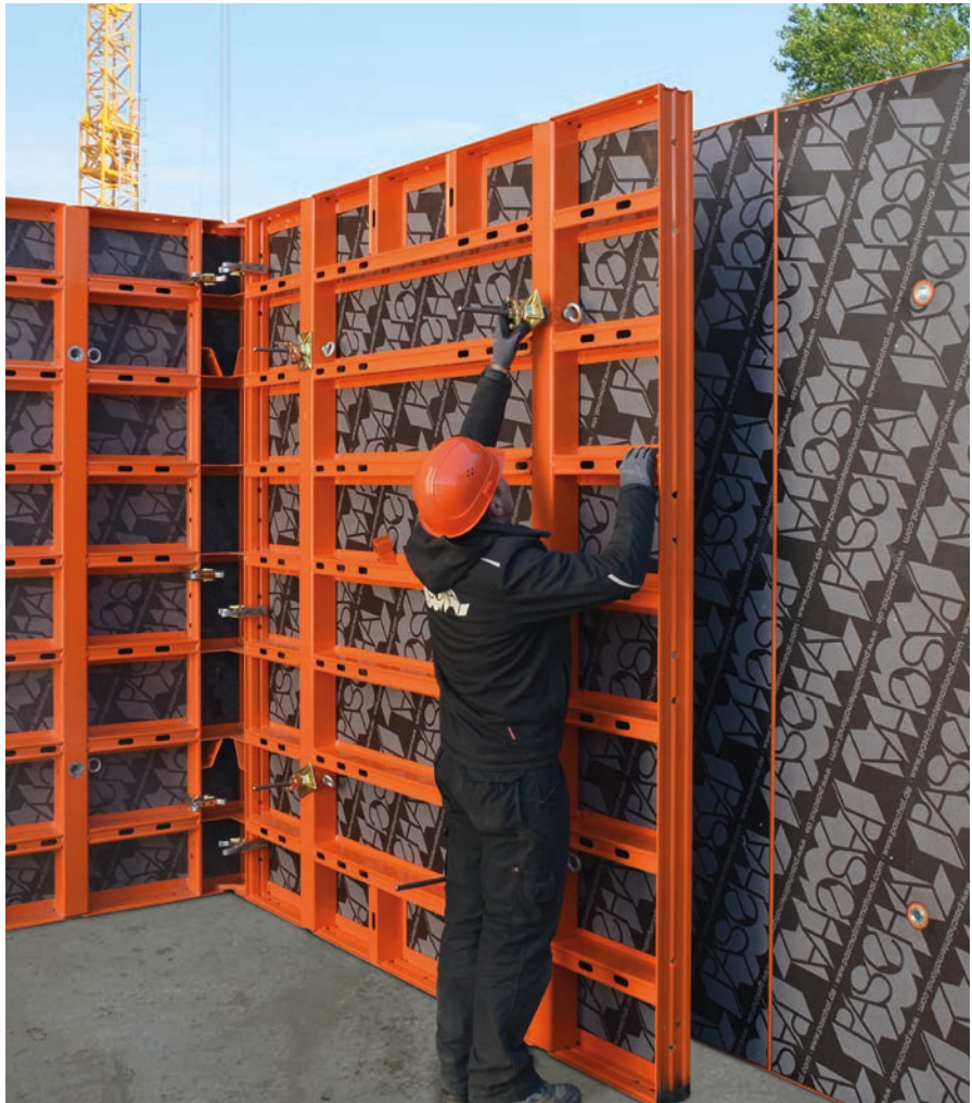
One-sided anchor technology makes the formwork anchors easy to operate by just one person
