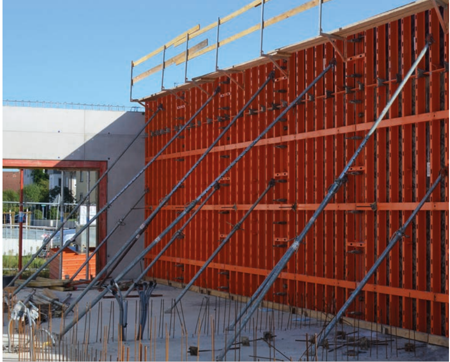
Building for production, D-Haslach; Fa. Singler Bau, D-Hofstetten
