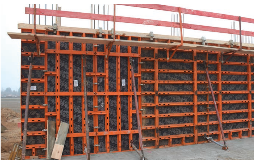
Parzival school, D- Karlsruhe; Weisenburger Bau GmbH
