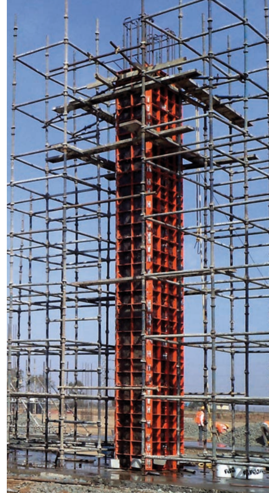
Angle column consisting of Modular panels and rigid 135° corners, suitable formed without expensive special formwork.
