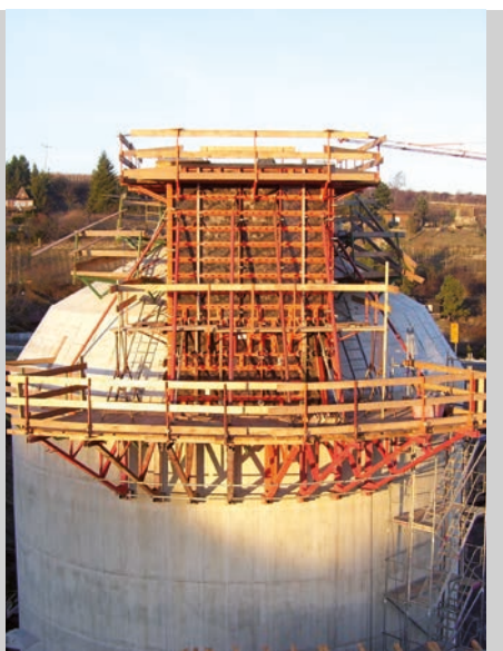
Sewage plant - Extension of the digestion tower, D-Rollsdorf; beton & rohrbau GmbH & Co.KG, D-Halle
