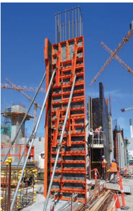
Waste incineration plant „Amager Bakke“, DK-Copenhagen; NCC, DK-Copenhagen
