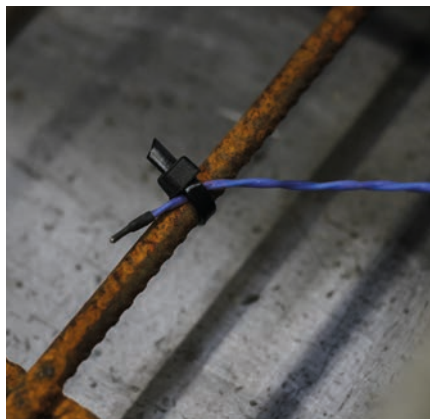
The sensor cable is attached directly to the reinforcement and connected to the radio transmitter.
