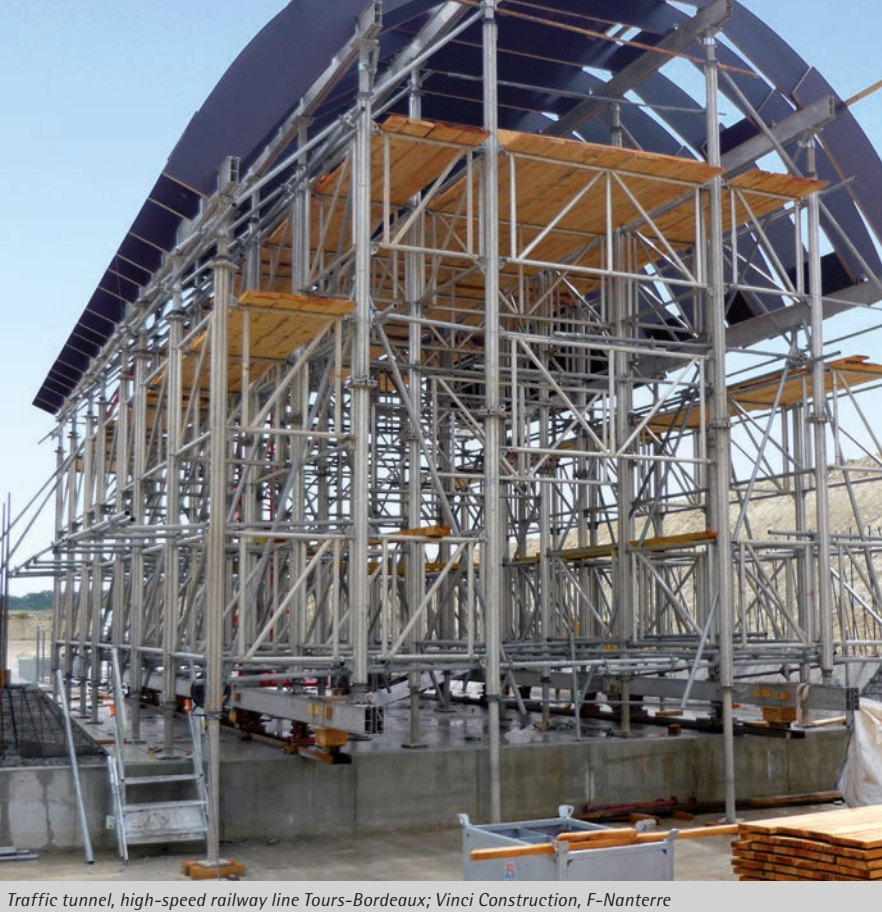
Traffic tunnel, high-speed railway line Tours-Bordeaux; Vinci Construction, F-Nanterre
