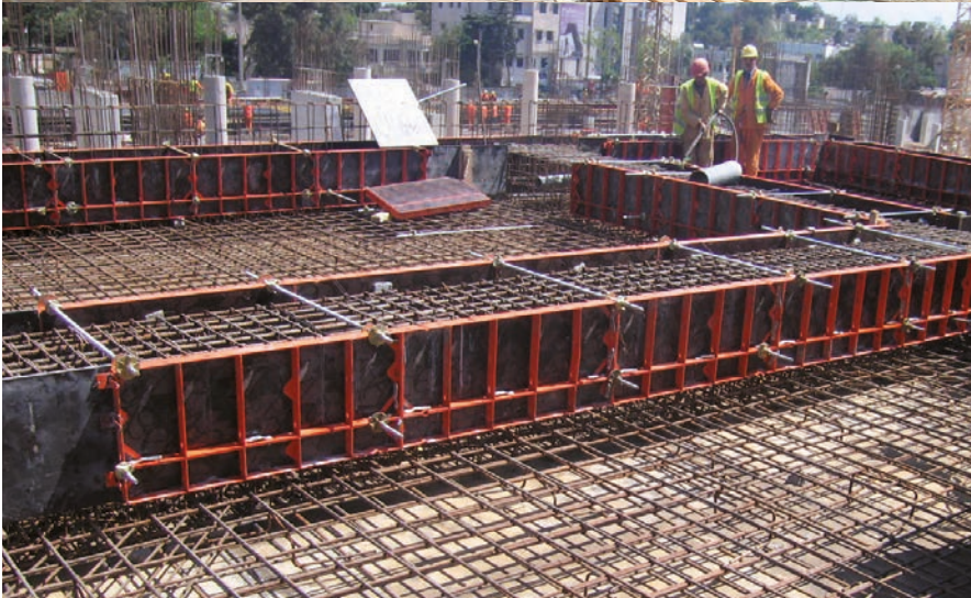
Medical faculty Algiers, DZ-Algiers ; Fa. Entreprise COSIDER-Construction, DZ-Dar El Beida, Algiers
