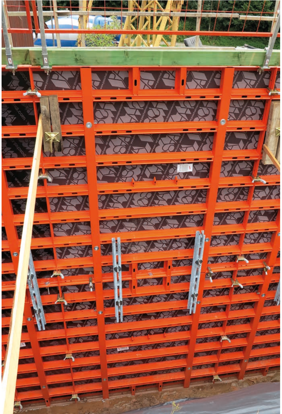
For single-sided anchoring, the tie rod together with the tube, the guide bushing and plate with ball-andsocket joint are turned into the clamping unit of the outer formwork.
