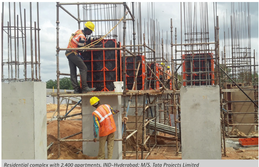
Residential complex with 2,400 apartments, IND-Hyderabad; M/S. Tata Projects Limited
