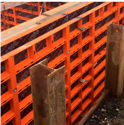
Unscrew the tie rod with the plate with ball-and-socket joint during dismantling.
