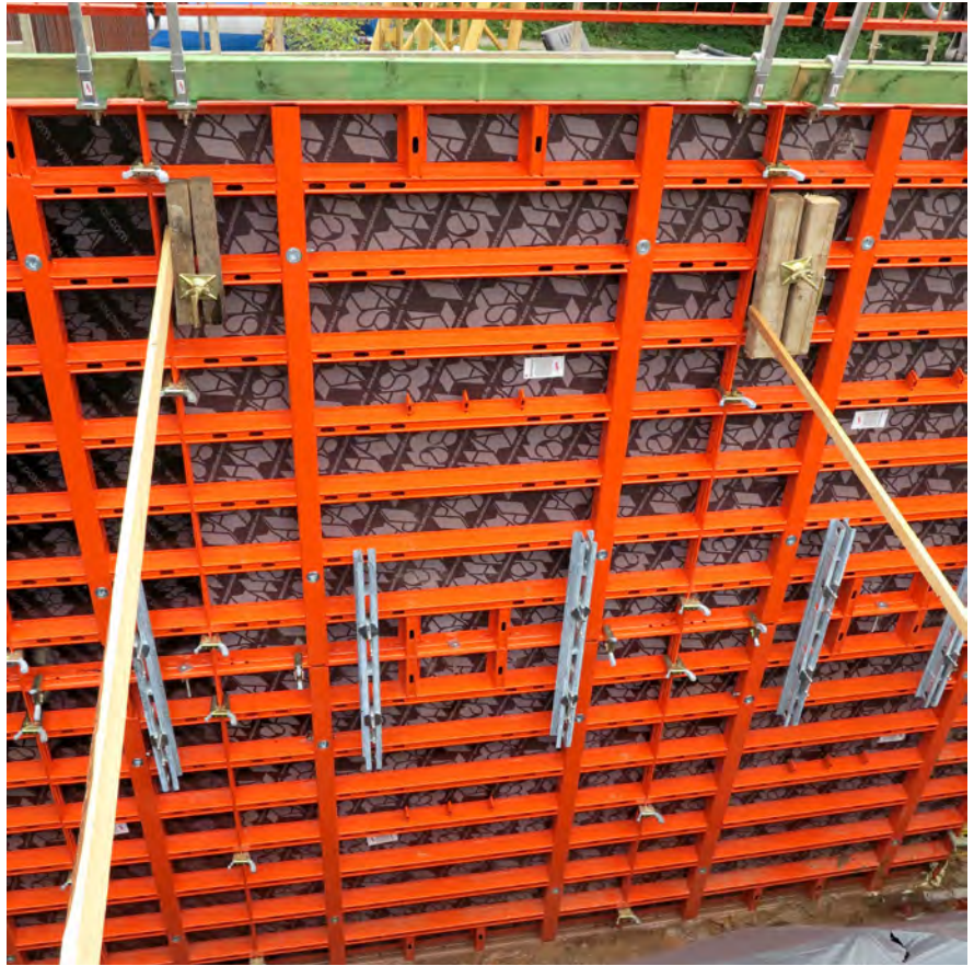
For single-sided anchoring, the tie rod together with the tube, the guide bushing and plate with ball-and-socket joint are turned into the clamping unit of the outer formwork.
